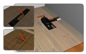
Measure the shower drain base position on the floor and mark this onto the relevant flooring. Using a jigsaw cut a hole in the plywood so that the shower drain base and shower drain connector will be exposed through the new floor.
