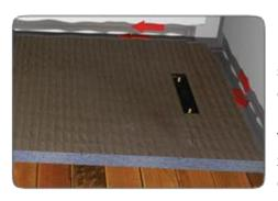
Using the Tanking Solution and a paintbrush, apply a thin layer of Tanking Solution to the Internal Corners of the shower tray, slightly bigger than the pencil line marked earlier. Place the waterproofing Internal Corners into the internal corners of the shower tray and push firmly into the Tanking Solution. Apply a further thin layer of Tanking Solution over the edges of the waterproofing Internal Corners.
